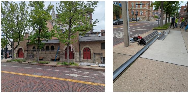
High winds in December caused damage to the church roof. Several of the ridge caps blew off. Additional damage was caused by high winds in March. Durable Slate Company fabricated and installed new ridge caps in May.
